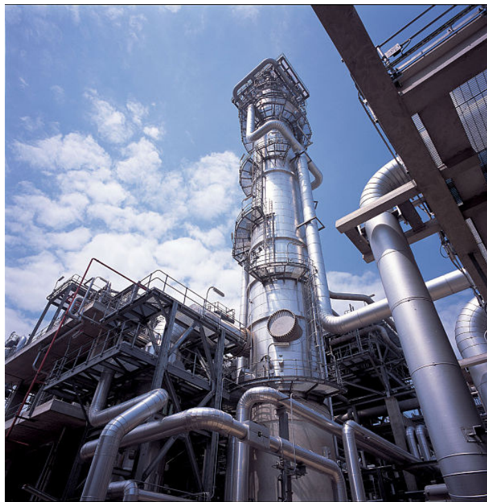
Figure 4: A typical column in a chemical plant
